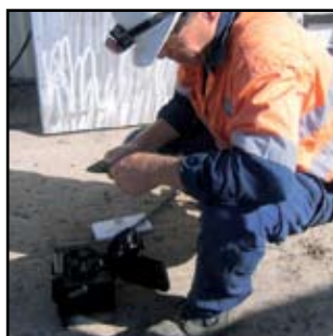
On-site MTP® splicing system
